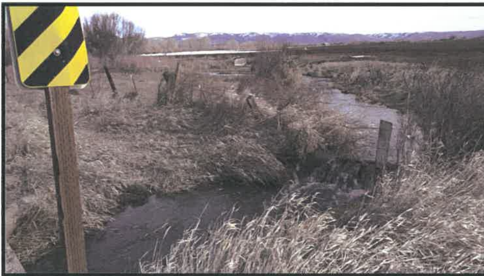
Figure 4. Photo of Coleman Creek at Culvert 3 looking northeast.
