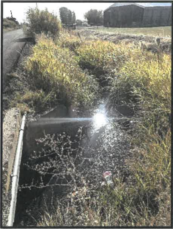
Figure 1. Photos of Coleman Creek Segment 2 looking downstream (south) from Culvert 1
