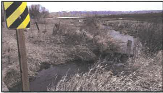
Figure 6. Photo of Coleman Creek at Culvert 3 looking northeast, likely impacted.
